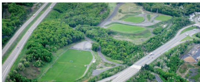
This regional park was constructed with FBC ash on the site of a former waste coal pile.
